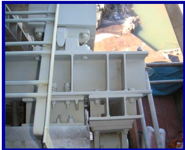
One of the spillway gates after coating – note the complex geometries.
