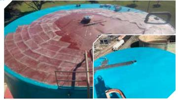
The surface was then primed with Plasmet ZF (red) ahead of using Epoxy Laminating Resin and quadriaxial fiberglass mat to laminate a composite fiberglass layer across the entire tank roof. The team then chose a suitable polyurethane topcoat to offer UV protection in a colour that matched the remainder of the tank. The client was extremely impressed with the final result and the quality assurance and will continue to work with Corrocoat US on future projects.
