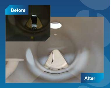
The tank was 7.5m long with a diameter of 1.91m. Access was provided through two off 600mm tank top manways and another at the bottom of the rear dish. The tank would be collecting acidic liquids, with the possibility of weak solvents, all at ambient temperatures. With this in mind, Polyglass VEF was the coating system selected for the job. Polyglass VEF is specifically designed to offer the corrosion in aggressive chemical environments and has a proven track record with road tankers
